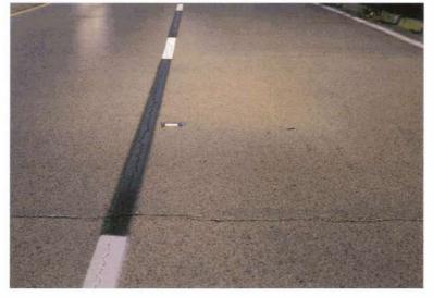
Roadway markers shine when struck by headlight beams to help drivers see the driving lane at night.
